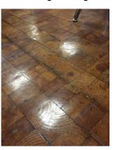
• The older piping under the Media Center has caused several other issues in the new flooring. The librarian reported that steam visibly penetrated the seams of the VCT tile during the first year of operation and the floor was extremely hot on the surface. This has been reported to have been resolved, but it needs to be determined whether possible damage has occurred to the adhesion of the VCT tile and underlayment.
