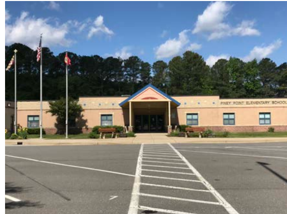
Piney Point Elementary
