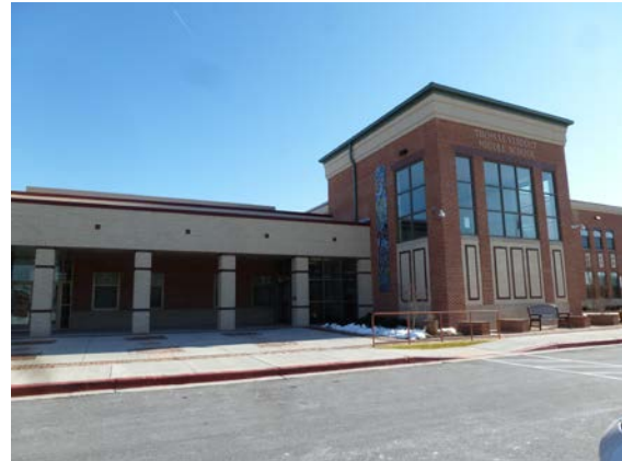
Thomas Viaduct Middle
