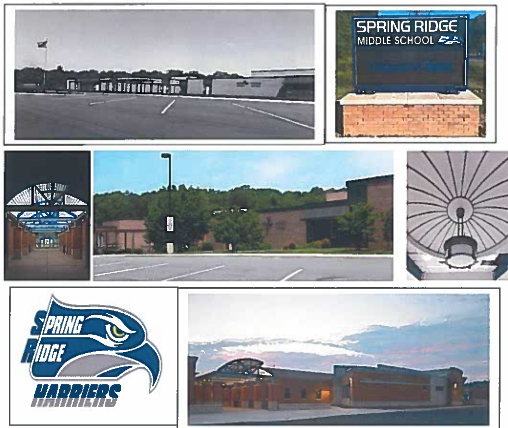
Spring Ridge Middle School Addition and Limited Renovation Completed August 2016
