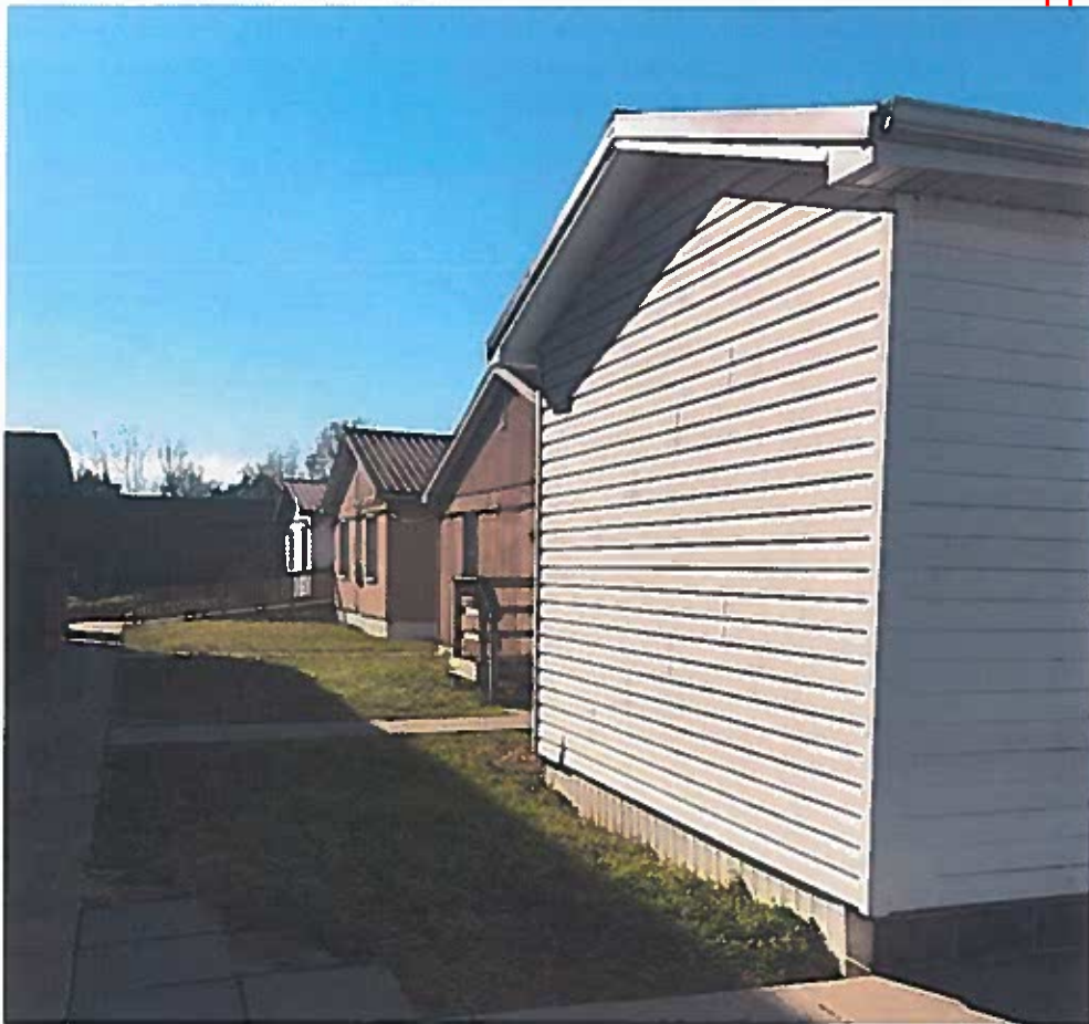
Nine temporary classrooms located behind the school
