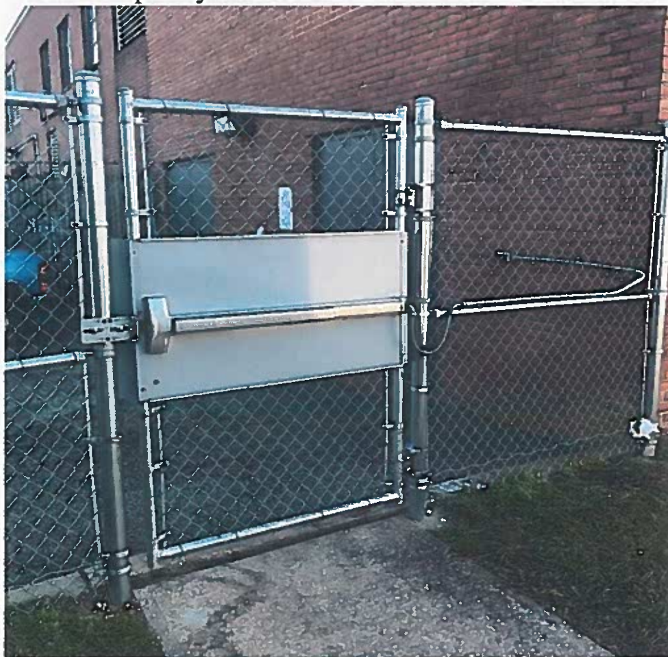
Additional security fencing installed around temporary classrooms
