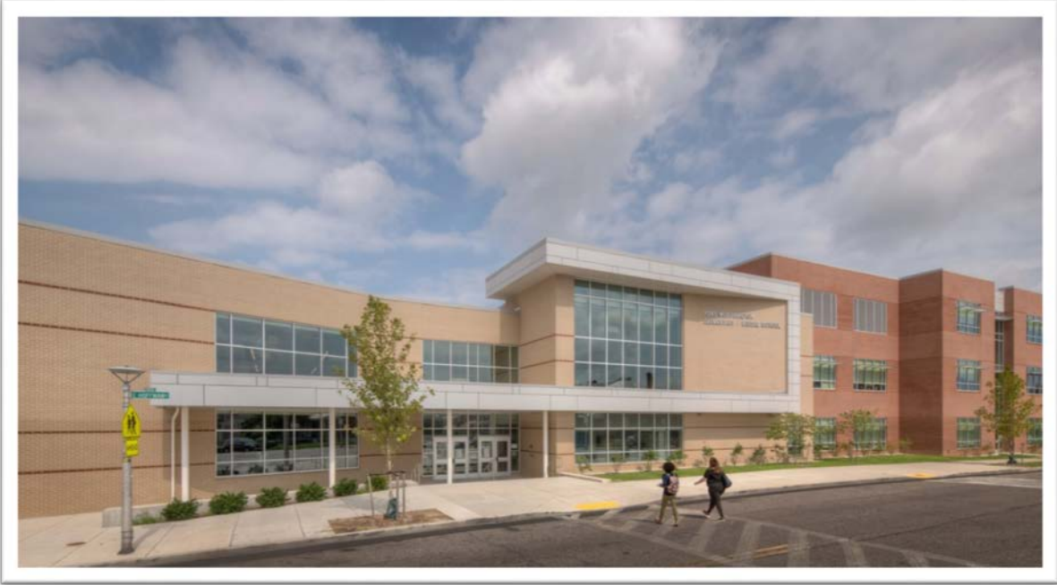
Figure 2. Fort Worthington Exterior
