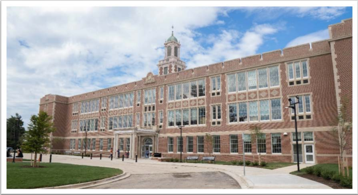
Figure 5. Robert Poole Building Exterior
