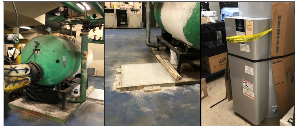
water heater installation at LOCKERMAN-BUNDY ES project status 50% CONSTRUCTION
