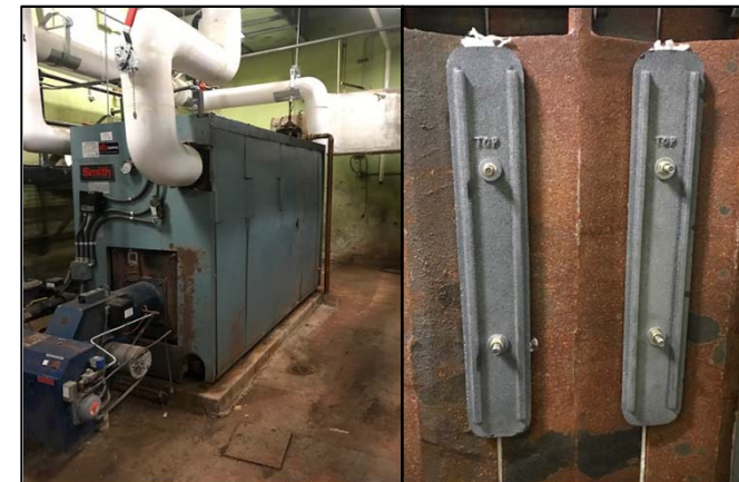
boiler section replacement at GWYNNNS FALLS ES project status OPERATIONAL
