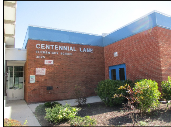
Centennial Lane Elementary
