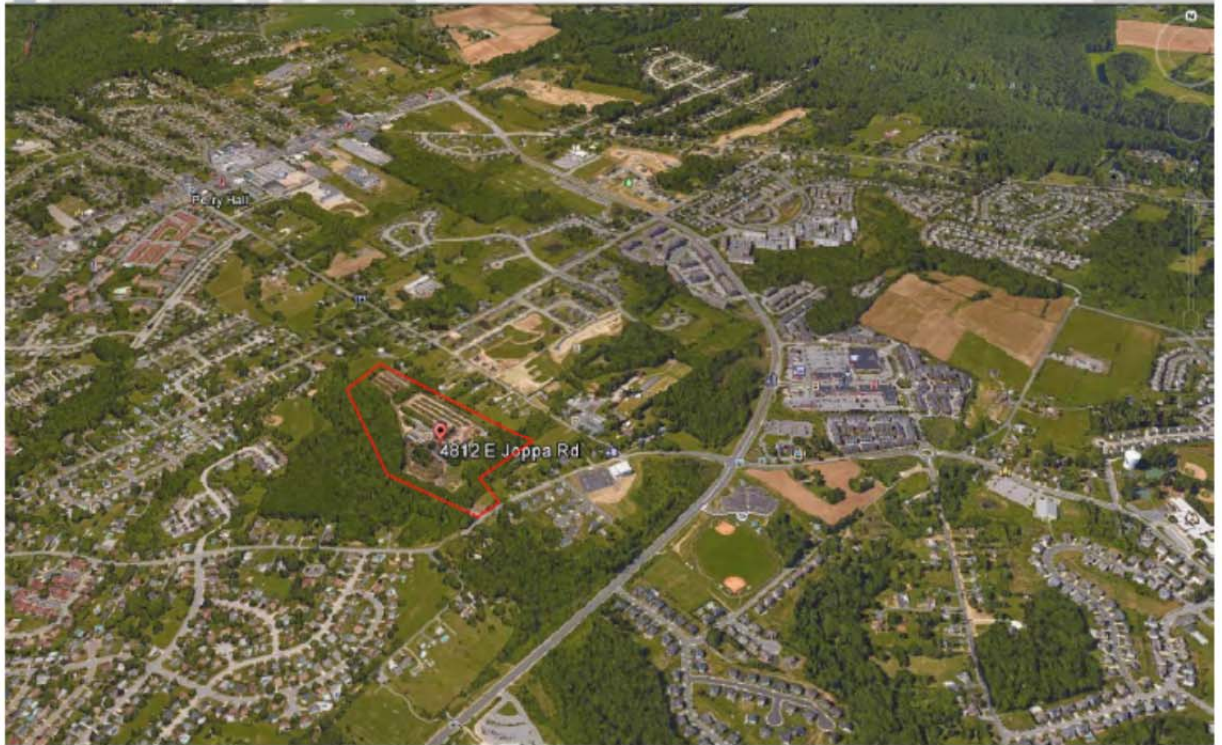
Northeast Area Elementary School – Bird's Eye View – Site Aerial
