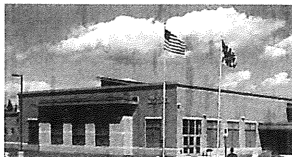
Figure A: Through the implementation of an EPC with NORESKO, BCPS will reduce water and energy consumption and lower operating costs while upgrading building infrastructure and improving the educational environment.
