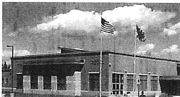
Figure A: Through the implementation of an EPC with NORESOCO, BCPS will reduce water and energy consumption and lower operating costs while upgrading building infrastructure and improving the educational environment.
