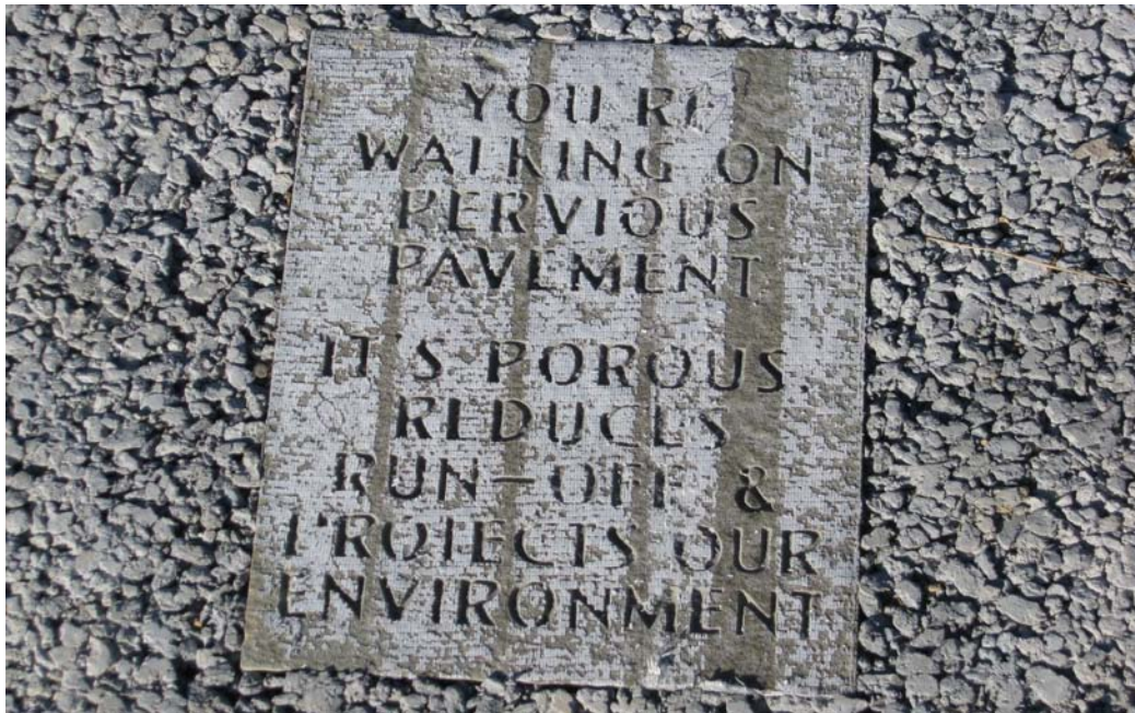
Pervious Pavement Linganore High School, Frederick County
