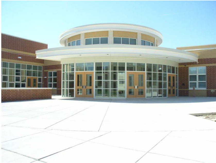
Francis Scott Key Middle School – Certified LEED Gold Montgomery County Public Schools
