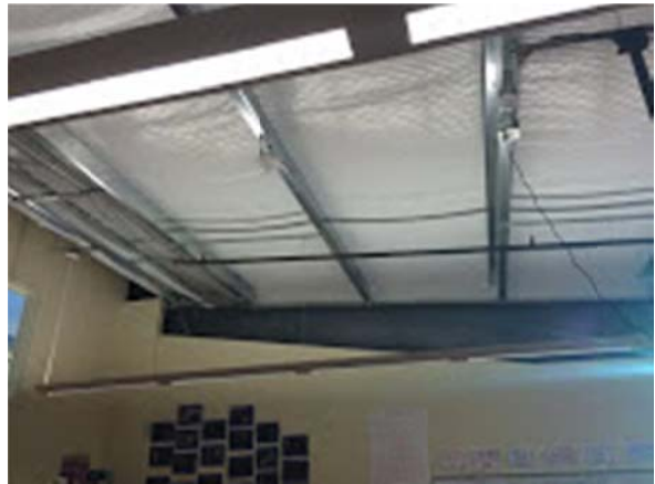
7. Second Floor Classroom Ceiling
