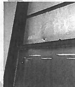
2 nd Floor Sash
