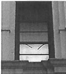
Exterior 2 nd Floor
