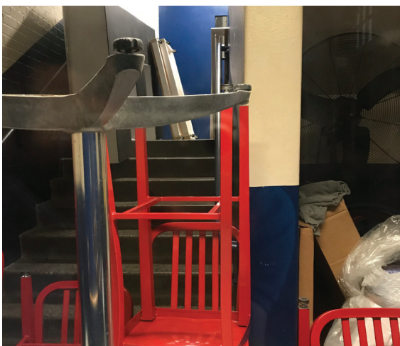
Stairway + water storage
