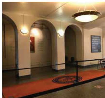
Bearing Wall at Tower Entry
