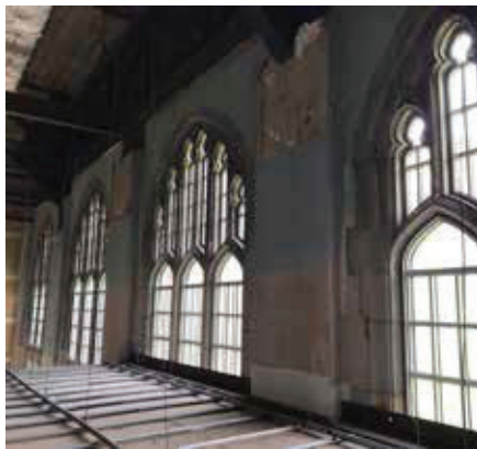
Auditorium Window Tracery Above Ceiling
