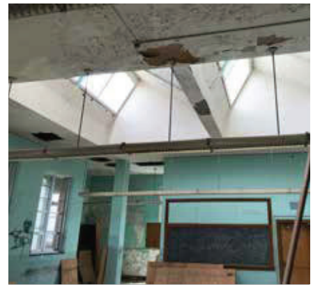
Fourth Level Skylights
