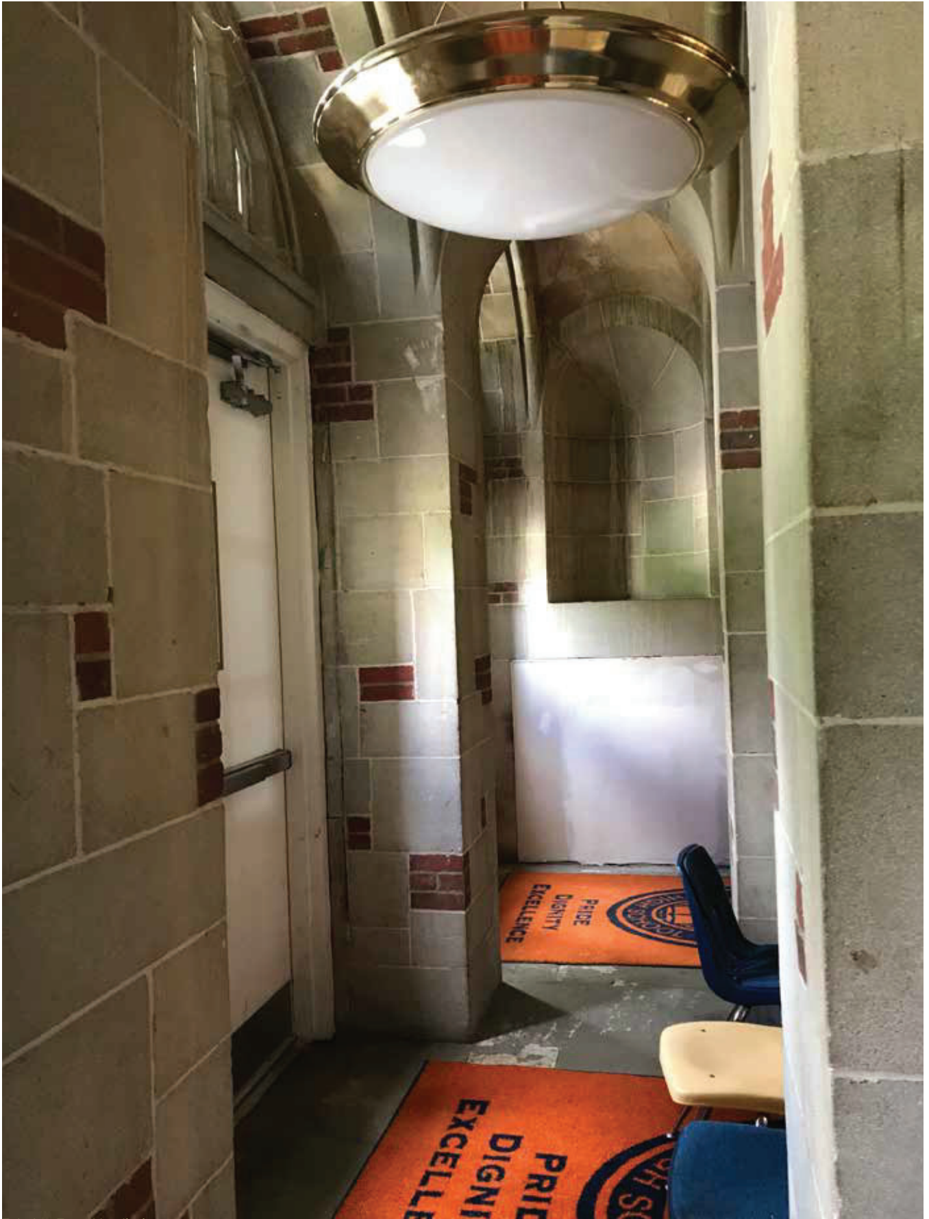
Existing Entry Vestibule
