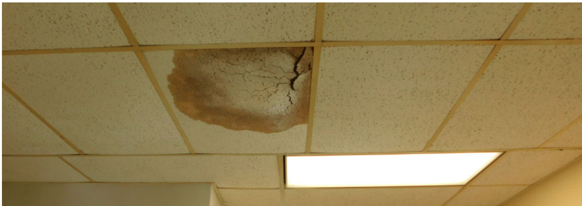
One of at least 2 signs of roof leak, 3 rd floor
